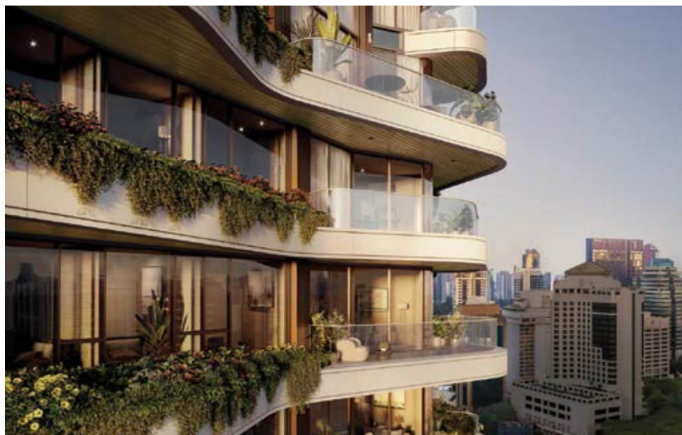
Park Nova's design incorporates a curved building exterior that mimics butterfly wings
