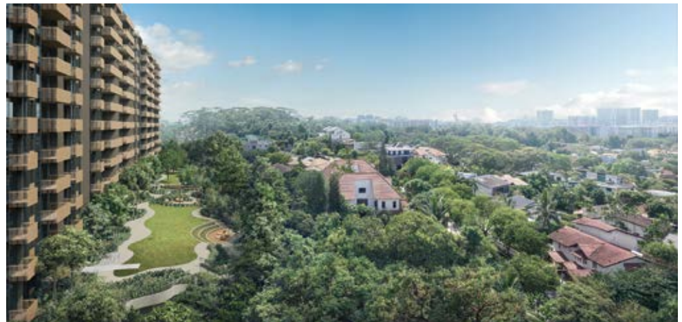
Units come with full-height glass facades and Juliet balconies, allowing residents to take in the views of the landed estate in Sunset Way
