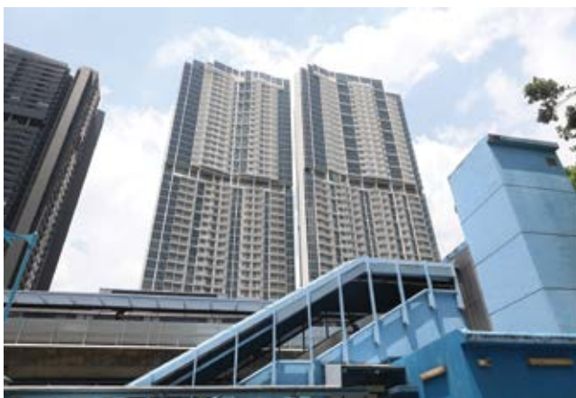
Queens Peak is directly linked to the concourse of Queenstown MRT Station
